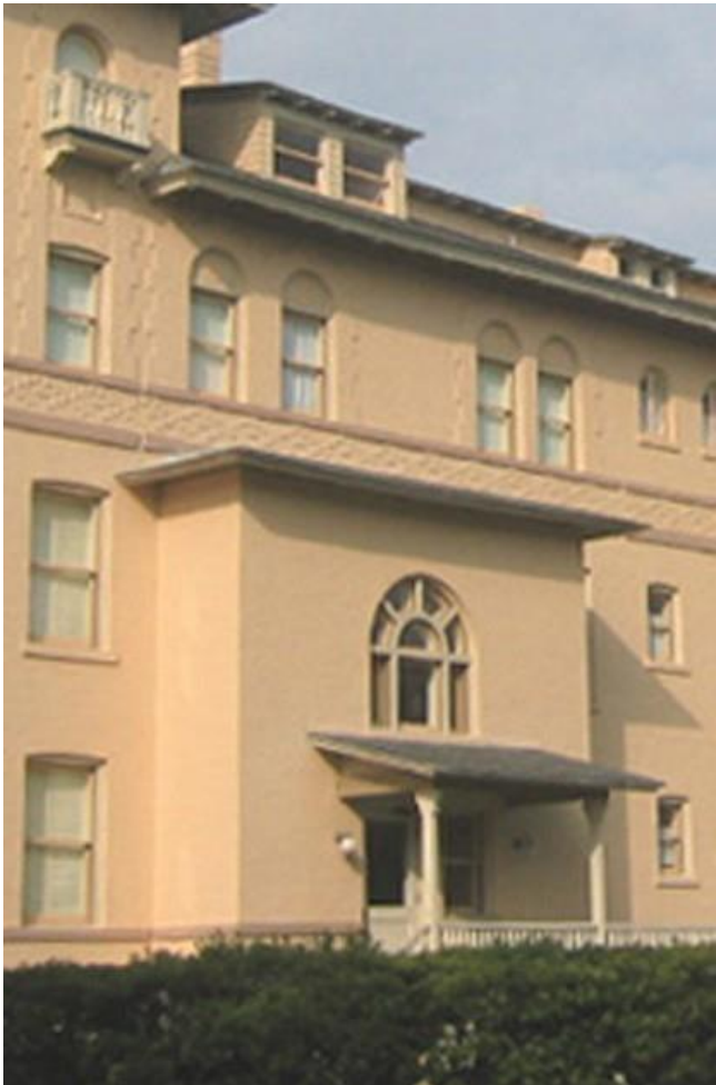
projected portals stopping one story below main roof capped with hipped roof
