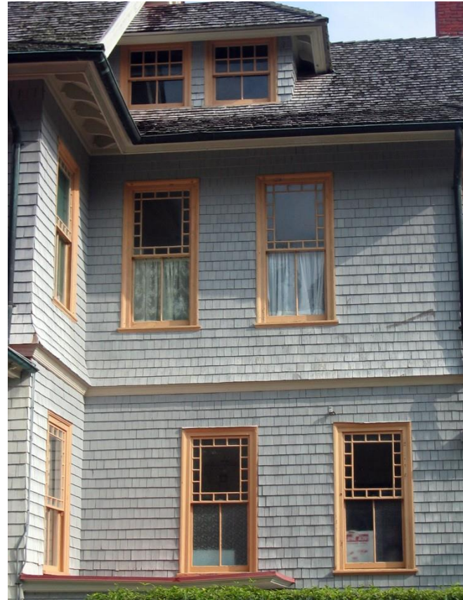
slight overhangs, either real or simulated with siding material, to avoid smooth wall appearance
