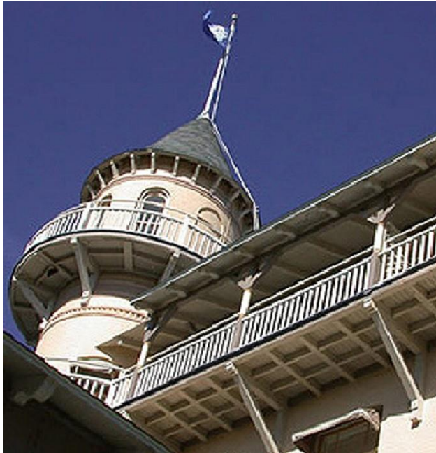
upper story porch with shed roof supported by brackets
